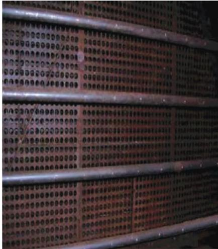
**8. In with a three-prong lance.** The new “three-prong” design added an additional AIG lance on each header where two had been used previously (Figure 7). Sidewall baffles were also added to improve ammonia mixing with the flue gas. *Courtesy: Cormetech*
