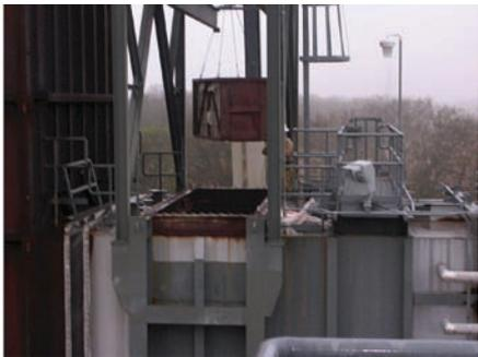
**4. Process improvement.** A sample tray was added to each of the new catalysts to ease access when collecting catalyst core samples for laboratory analysis. Drilling of the catalyst to collect a sample is no longer required. *Courtesy: Cormetech*
