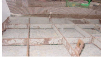
a. Removal of ash
